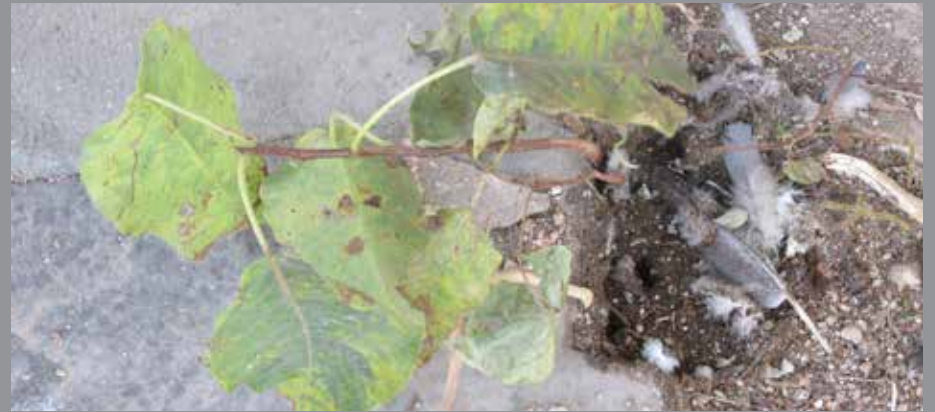
Fig 35 : Vegetation Ingress in floor
