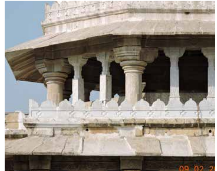
Fig 45: View showing replaced chajja at Rana Amar Singh I chattri
