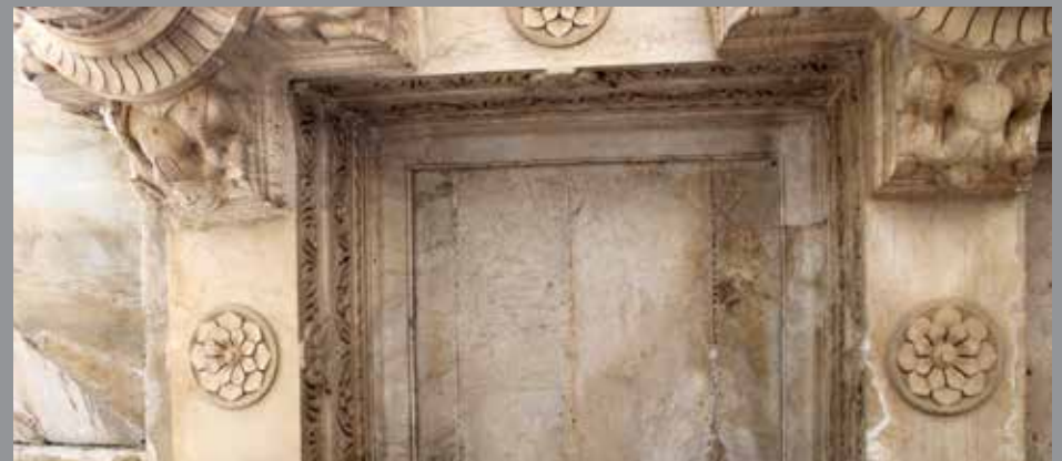
Fig 20: Calcination and flaking of stone surface
