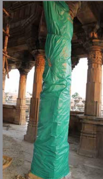
Fig 25: Covering the surface with plastic for 24 hr and then remove the plastic to let it dry completely
