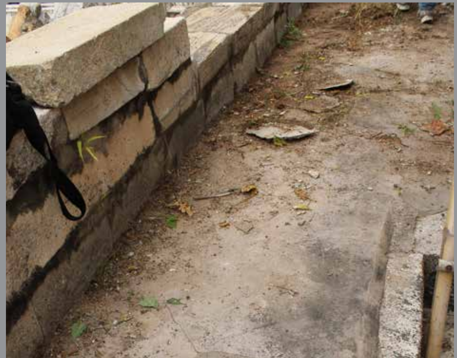
Fig 55 : Damaged flooring layer Rana Amar Singh I Chattri
