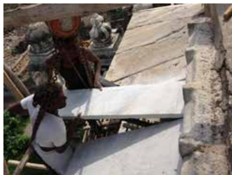
2.5.2– View of Fixing of Chajja for Level I – Work in Progress
