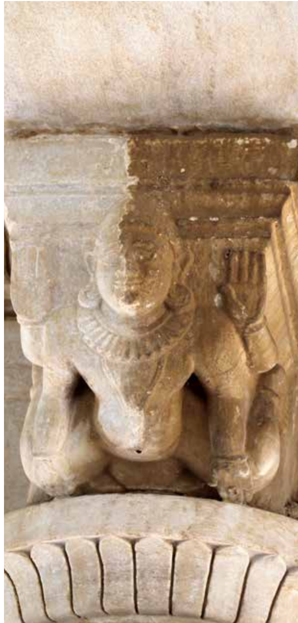
Fig 29: Before and After image of Calcination on stone surface - Rana Sangram Singh II chattri
