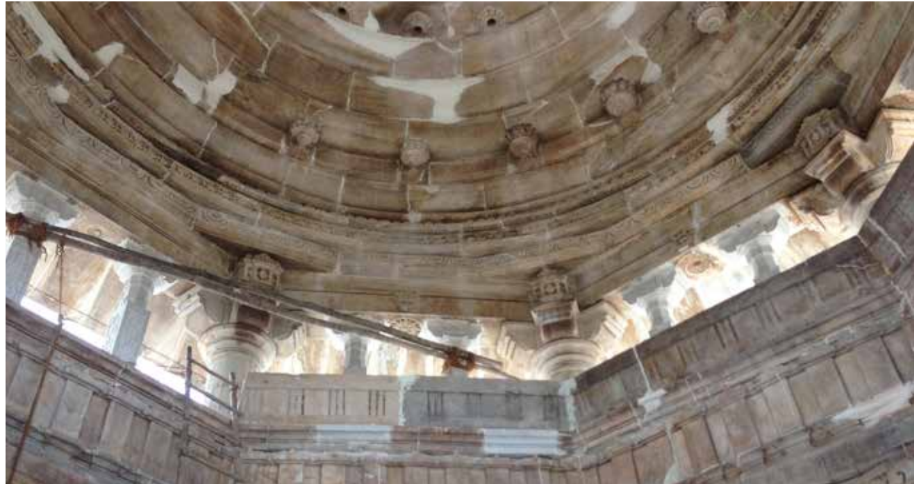
Fig 52 : View of patches of corbelling finished with lime and Jinki paste
