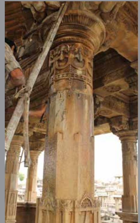
Fig 26: Remove the clay pack by washing the surface with water and scrubbing with brush.
