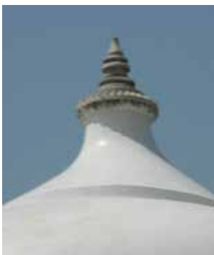
2.5.1 – Close view of the lime plaster and the Kalash on dome
