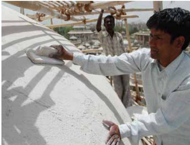
Fig: 56d: View of the finishing being given to lime and jinki quote
