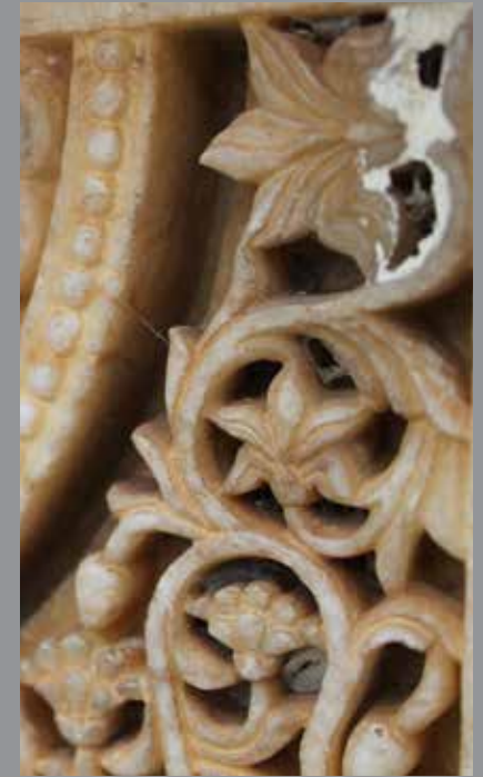
Fig 50 : Growth of micro organism in carving
