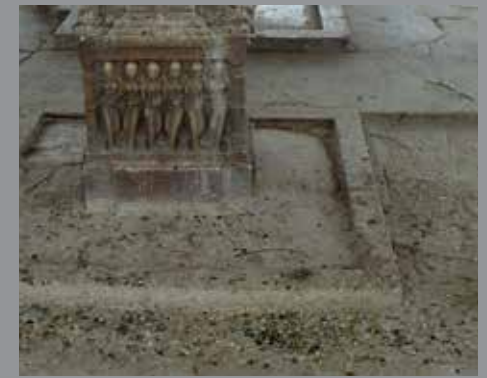
Fig 19: Bird dropping causing deterioration
