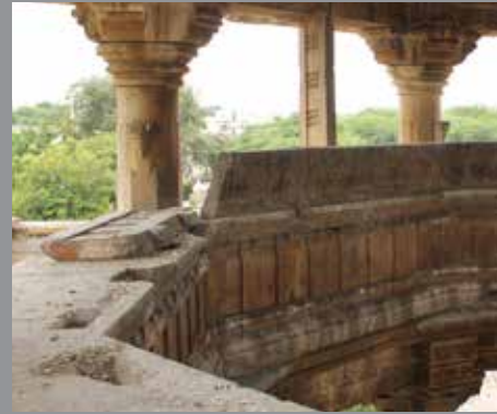
Fig 40 : View of broken parapet at level II
