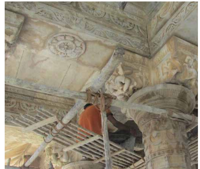
Fig 22b : View of the column, capital and beam of Rana Amar Singh I chattri after cleaning
