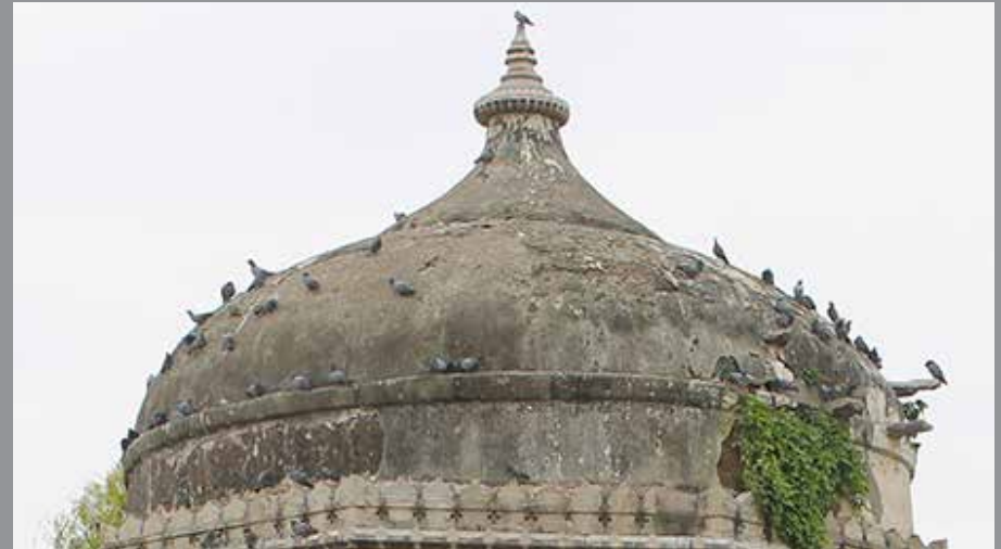
Fig 54: Deteriorating layer of lime plaster over the dome.
