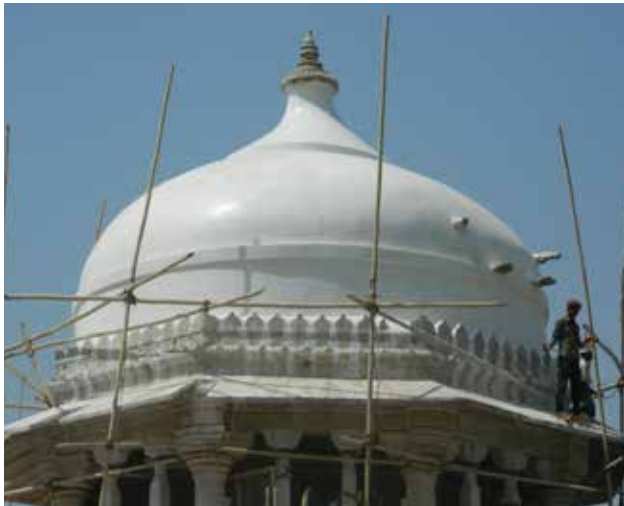
Fig: 56e: View of the dome after completion of dobara and nikhalas
