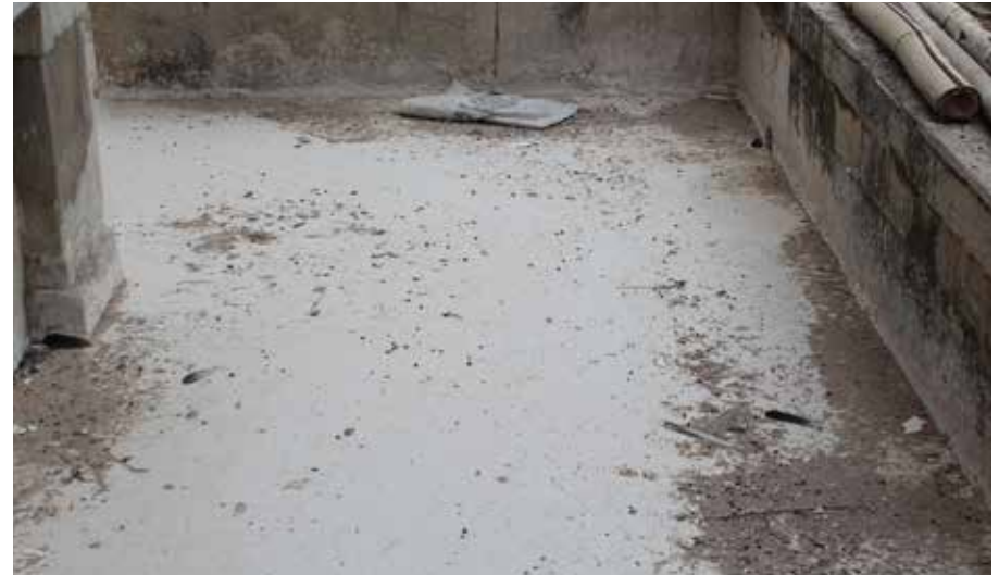
Fig: 57: View of the lime terracing redone
