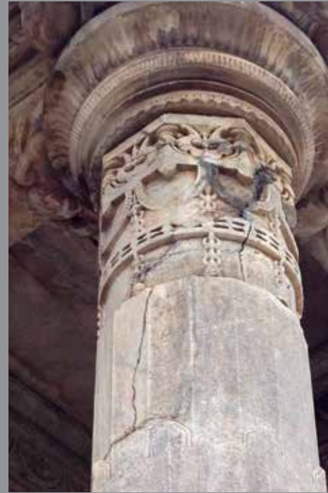
Fig 49: Crack in the column caused by undue movement of stone members
