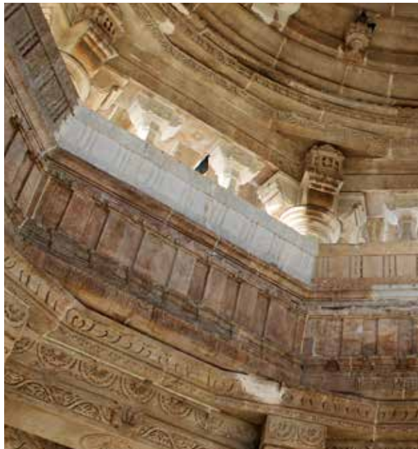
Fig 46: View of the parapet section reinstalled
