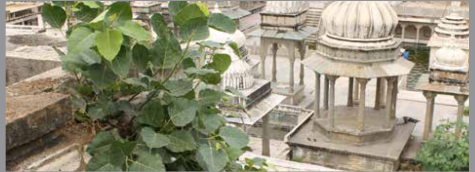
Fig 34 : Vegetation Ingress in Parapet joints
