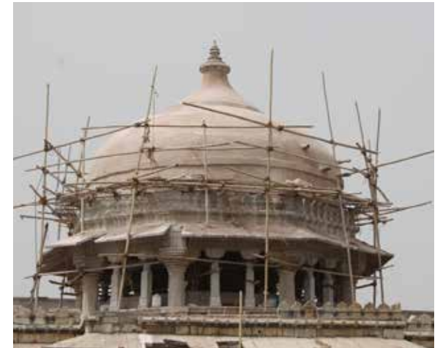
Fig: 56c: Surface of dome left for drying before applying lime and Jinki
