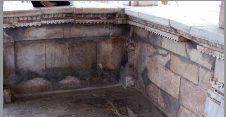
Fig 51 : Visible patches of past repair in cement
