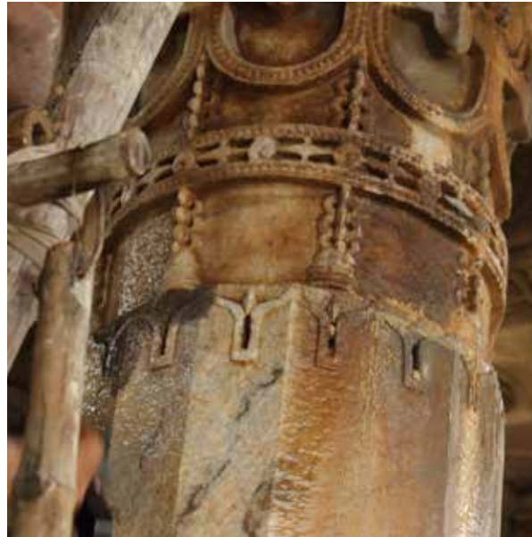
Fig 21 : Rana Amar Singh I stone surface before cleaning
