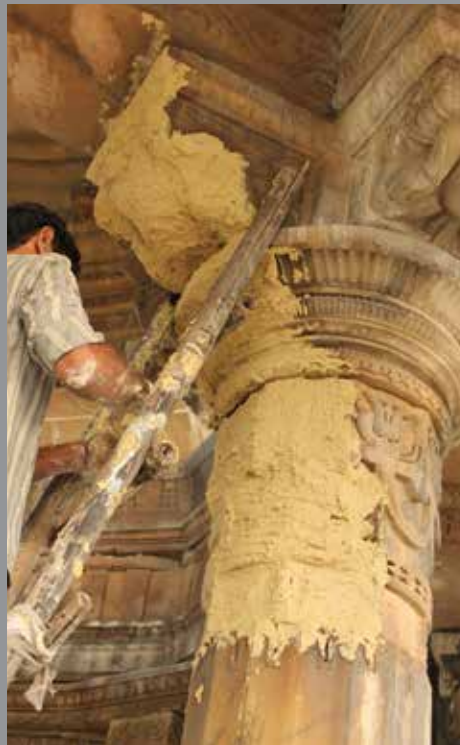
Fig 24: Application of clay pack to the surface
