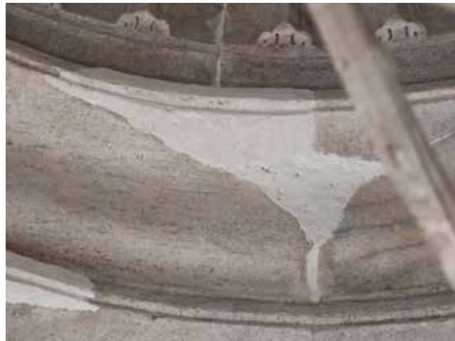
Fig 53: Close view of lime and Jinki filling to match the design
