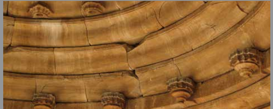
Fig 42 : Structural crack in the corbelling of the dome
