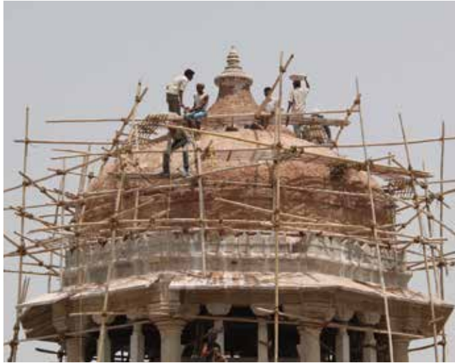
Fig: 56a: View of the layer 1 of restoration work using Lime, Surkhi and sand
