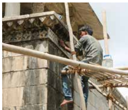
2.5.3 – View of Cleaning process in progress for plinth base
