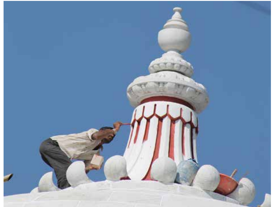
Fig: 58: Image showing Kalash after restoration and finished using gheru
