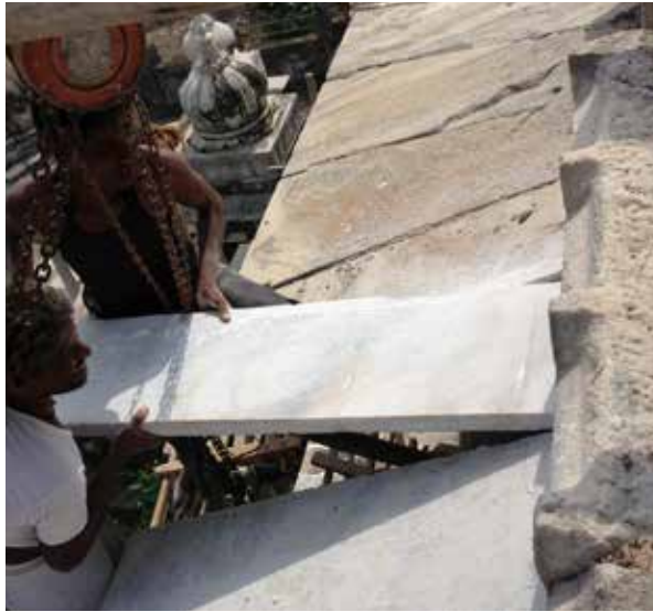
Fig 44: Fixing of Chajja in progress - Rana Amar Singh I chattri
