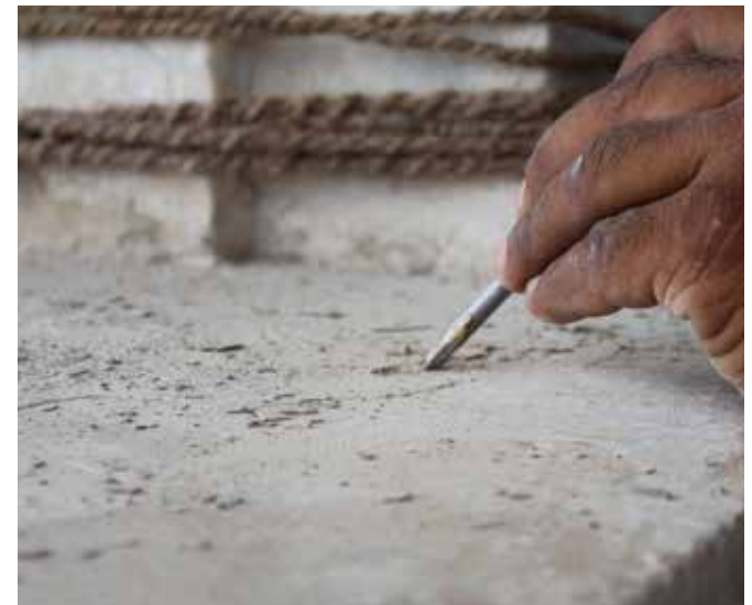
Fig 31: View showing cleaning of calcination on stone surface - Rana Sangram Singh II chattri
