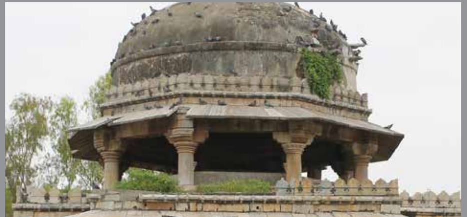
Fig 36 : Vegetation Ingress on the dome surface
