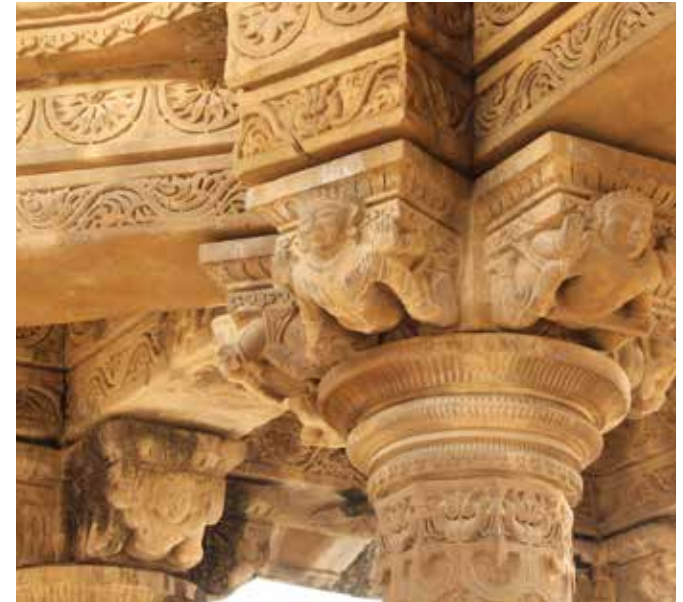
Fig 22a : View of the column, capital and beam of Rana Amar Singh I chattri before cleaning
