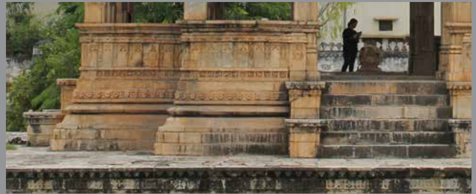
Fig 17: Flaking of stone surface
