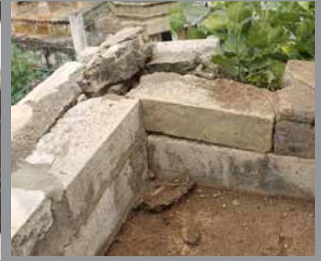
Fig 41 : Broken parapet Wall at Level II
